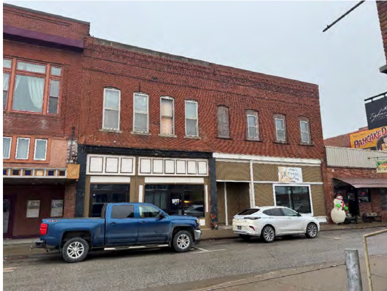
Existing Building Exterior
